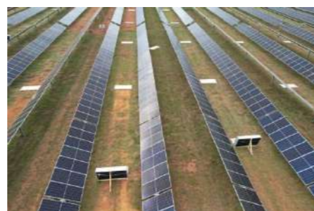
Texas Project Site (407.7MW)
